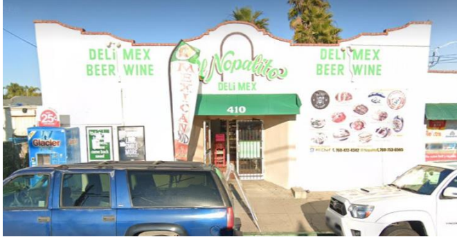
Figure 36: Spanish Eclectic commercial building in the Eastside neighborhood.
